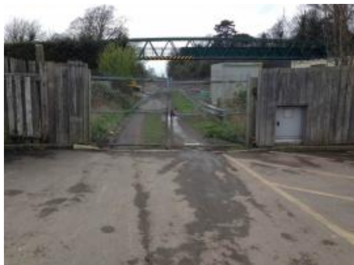
Photograph 8 – Land to the Rear of High Street Car Park
