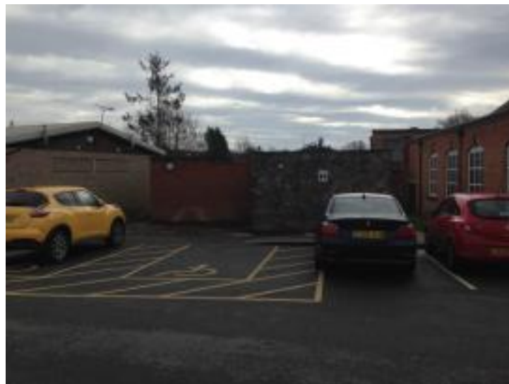
Photograph 18 – Public Toilets at King Street Car Park
