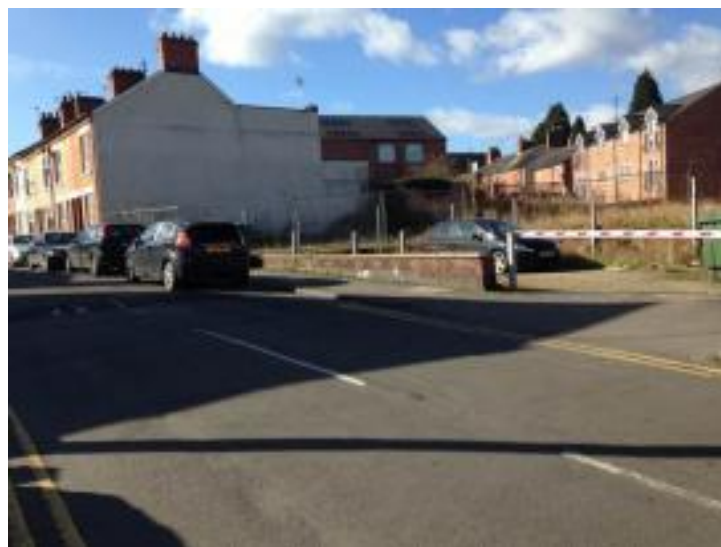
Photograph 1 – Latimer Street Site
