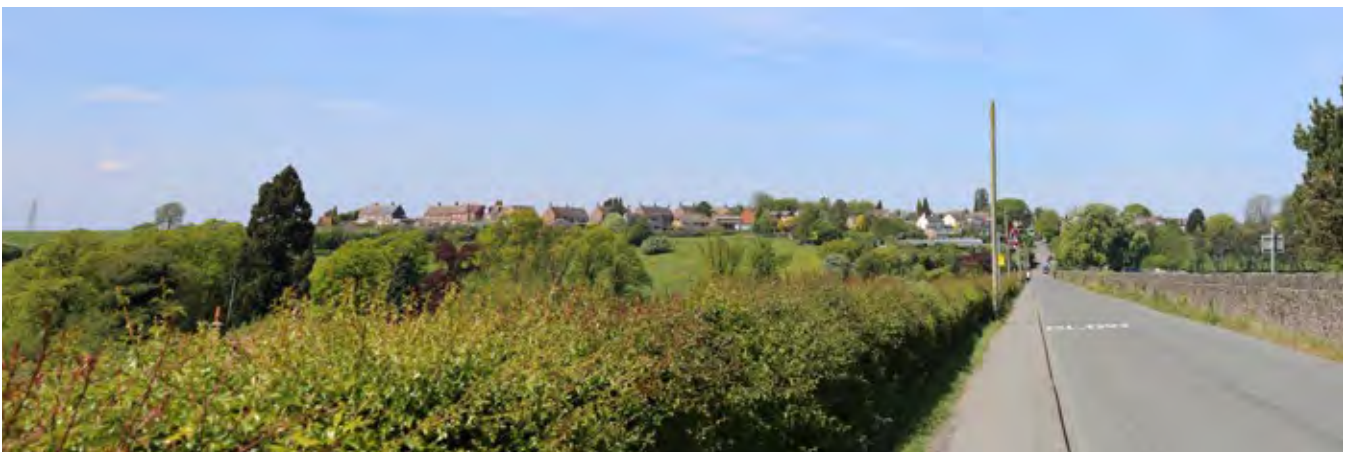
View of settlement edge from Reservoir Road
