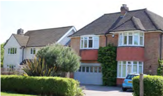
2 storey dwellings on Chavney Road
