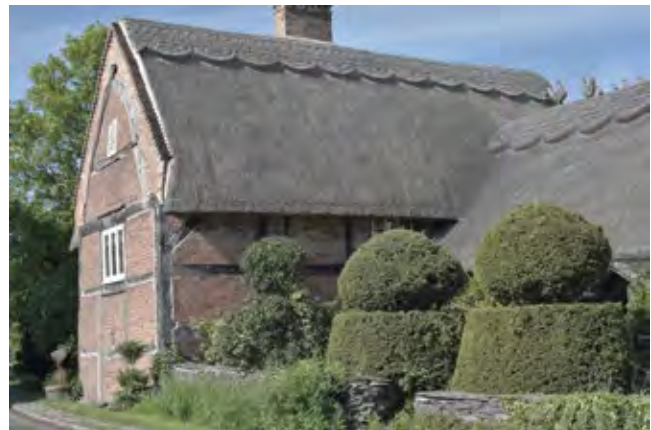
Traditional thatched roof and red brick materials
