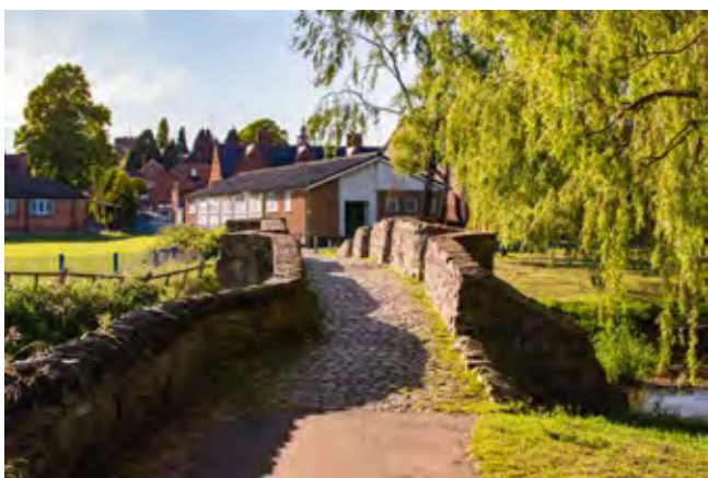
Approach to village over Packhorse Bridge
