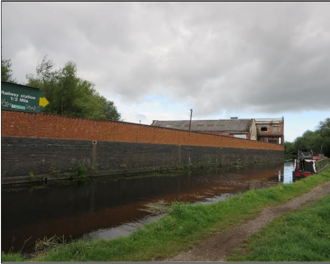
View of the site from the Grand Union Canal towpath
