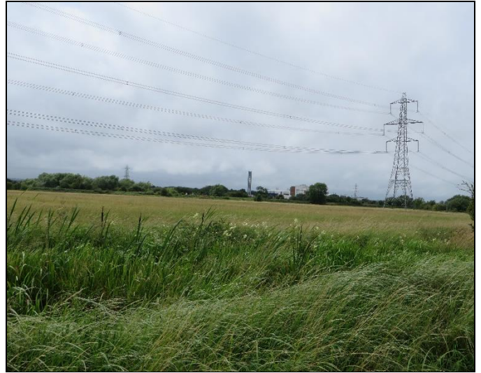
Pylons and overhead lines are prominent skyline features within the site
