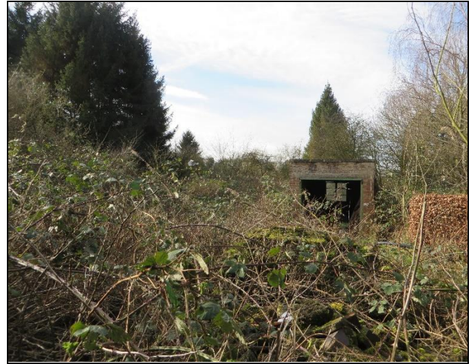
Surrounding land appears neglected and overgrown
