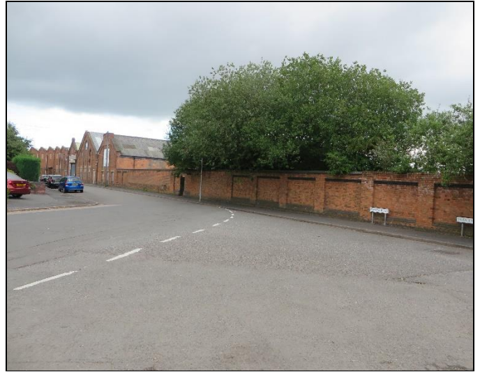
The site is enclosed by red brick walls and vegetation
