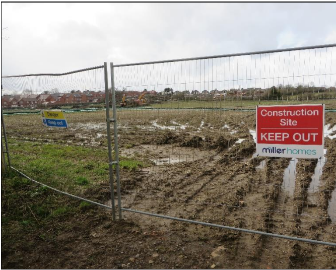
View of construction activity on the site
