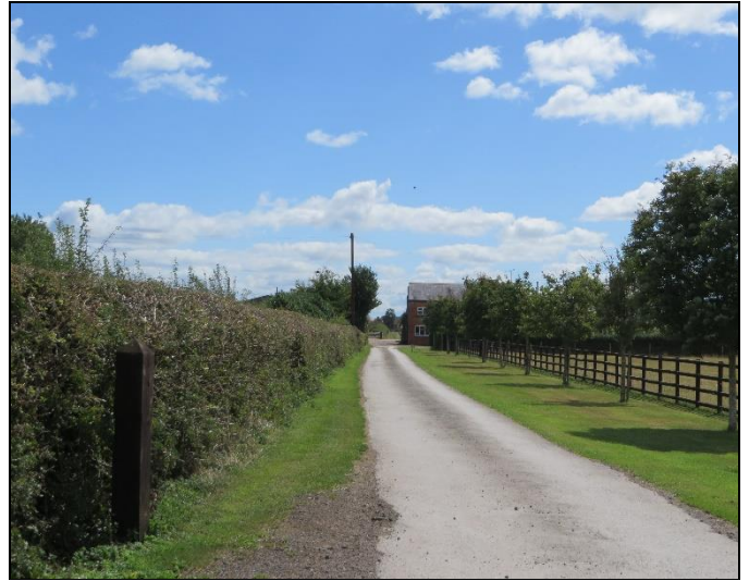
The entrance to the site from Hawthorn Road. Mature vegetation partially screens views from this direction.
