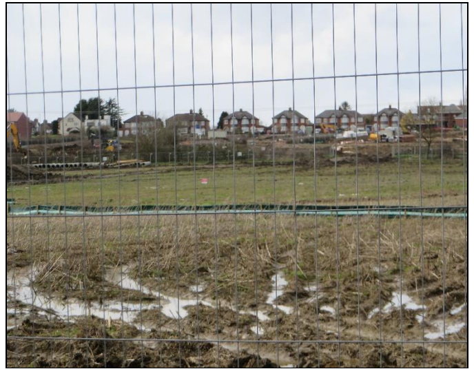
Existing houses in Sibley overlook the site
