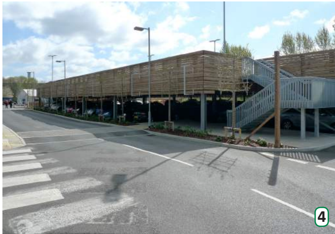
Decked car parking to increase efficient use of land and allow other parts of the site to be developed
