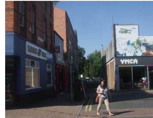
Opportunity to improve access to Queen's Park via Devonshire Lane
