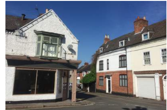
Character buildings with continuous frontages
