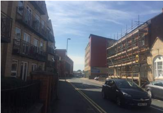
One way working on Woodgate
