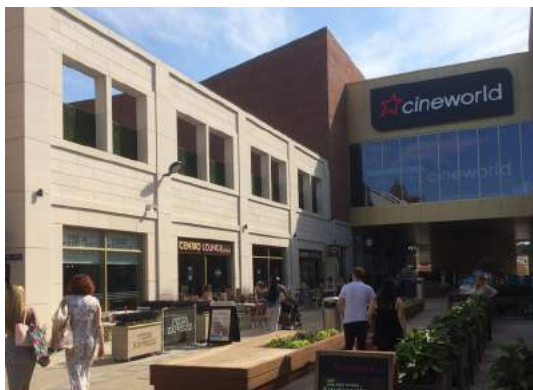
New Cineworld complex at Baxter Gate
