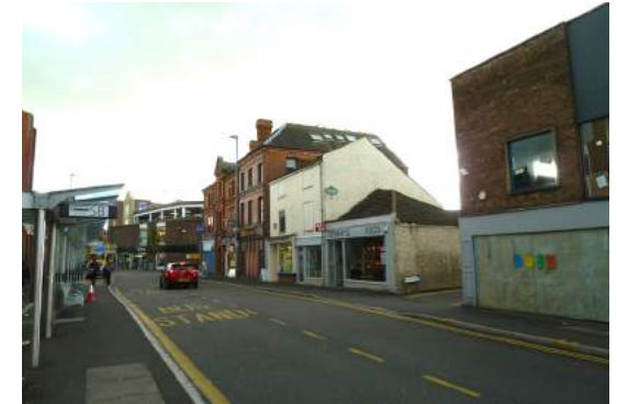
Inconsistent building form along The Rushes
