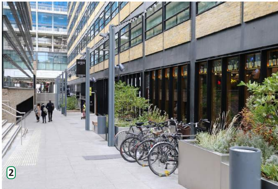
An active frontage could be created along the Devonshire Lane facade - animating the route to Queen's Park.
