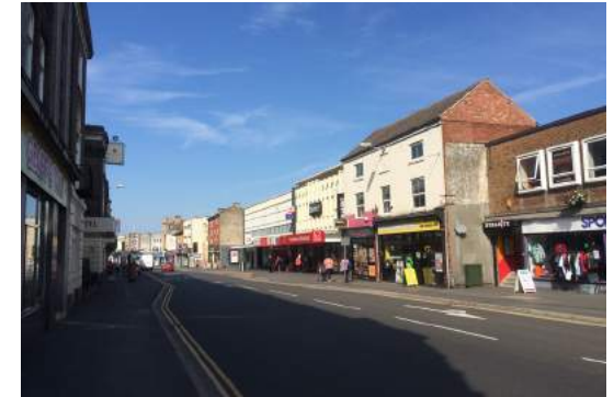
Poor quality buildings along High Street
