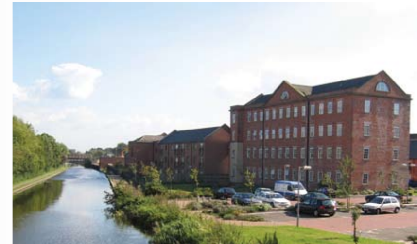
Former Towles Factory
