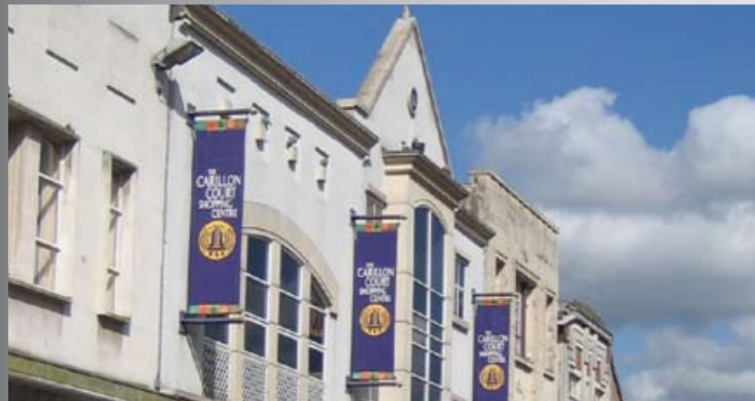
Carillon Court Shopping Centre
