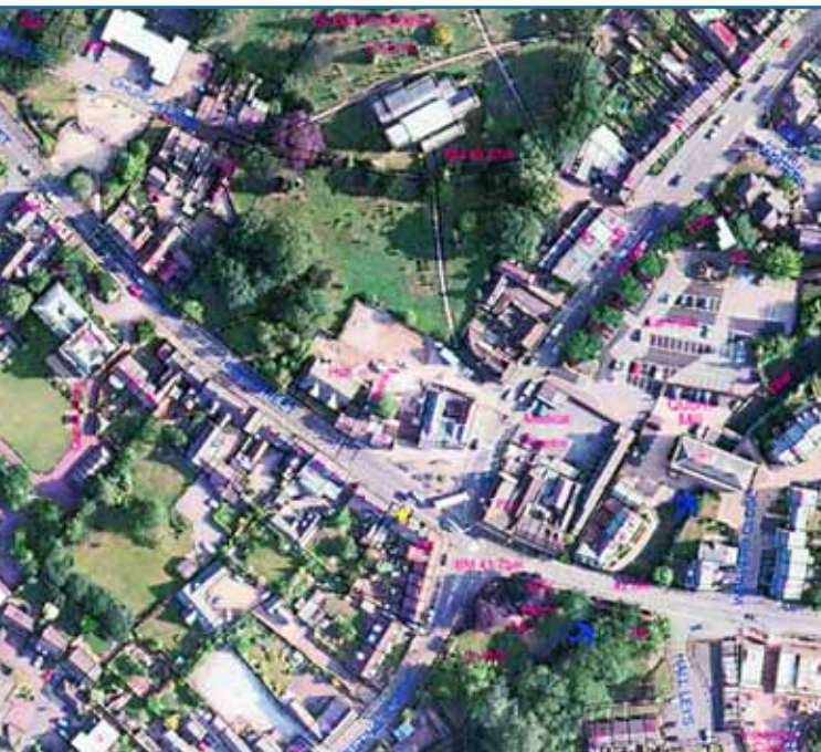
Aerial view above Quorn Cross
