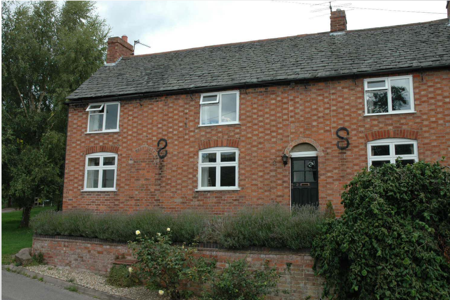
Flemish bond brickwork
