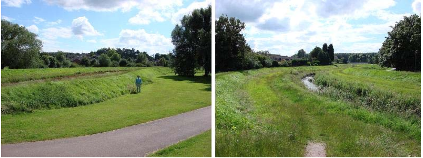
Plate 4.7 (left hand image) shows the height of the embankments along the Burleigh Brook at Thorpe Acre (view is to the southwest); note person for scale; and Plate 4.8 (right hand image) shows a typical view of the two-stage channel between the flood embankments.
