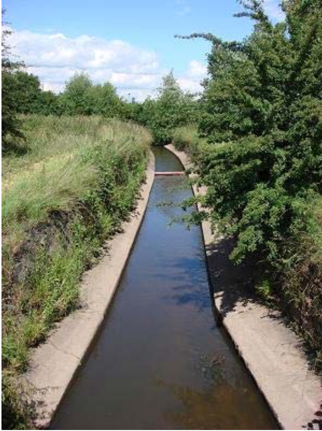
Plate 4.5 (left hand image) shows the downstream view (eastwards) along the Burleigh Brook from Canalside – note concrete bed; and Plate 4.6 (right hand image) shows the upstream view – note encroaching development and confined artificial channel and banks.
