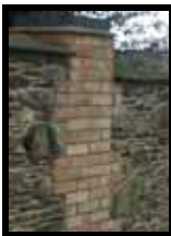
Granite walls with brick posts
