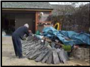
Sorting roof slates
