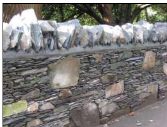
Newly built dry stone wall, Brand Hill
