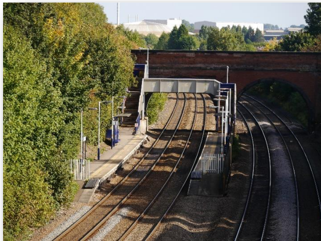
Figure 15: Barrow upon Soar Railway Station
