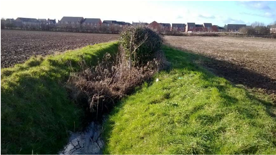
Image EDP A3.4: Running water ditch adjacent to hedgerow H6.
