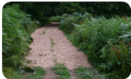
Step 1: Prepare Surface
