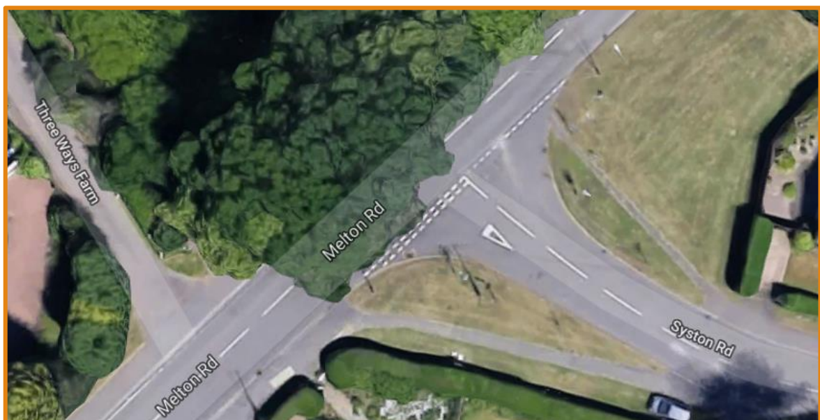
Figure 16: Syston Road/Melton Road T-junction
