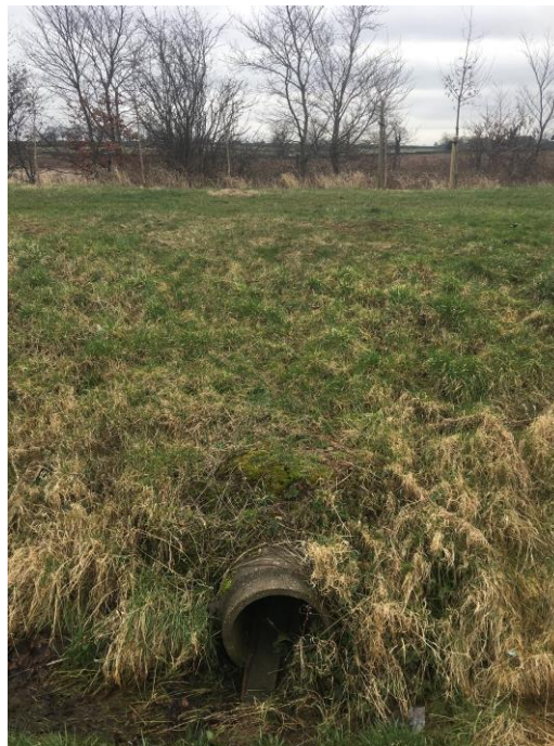
Figure 2-3: Development outfall looking from outside the site on the western boundary
