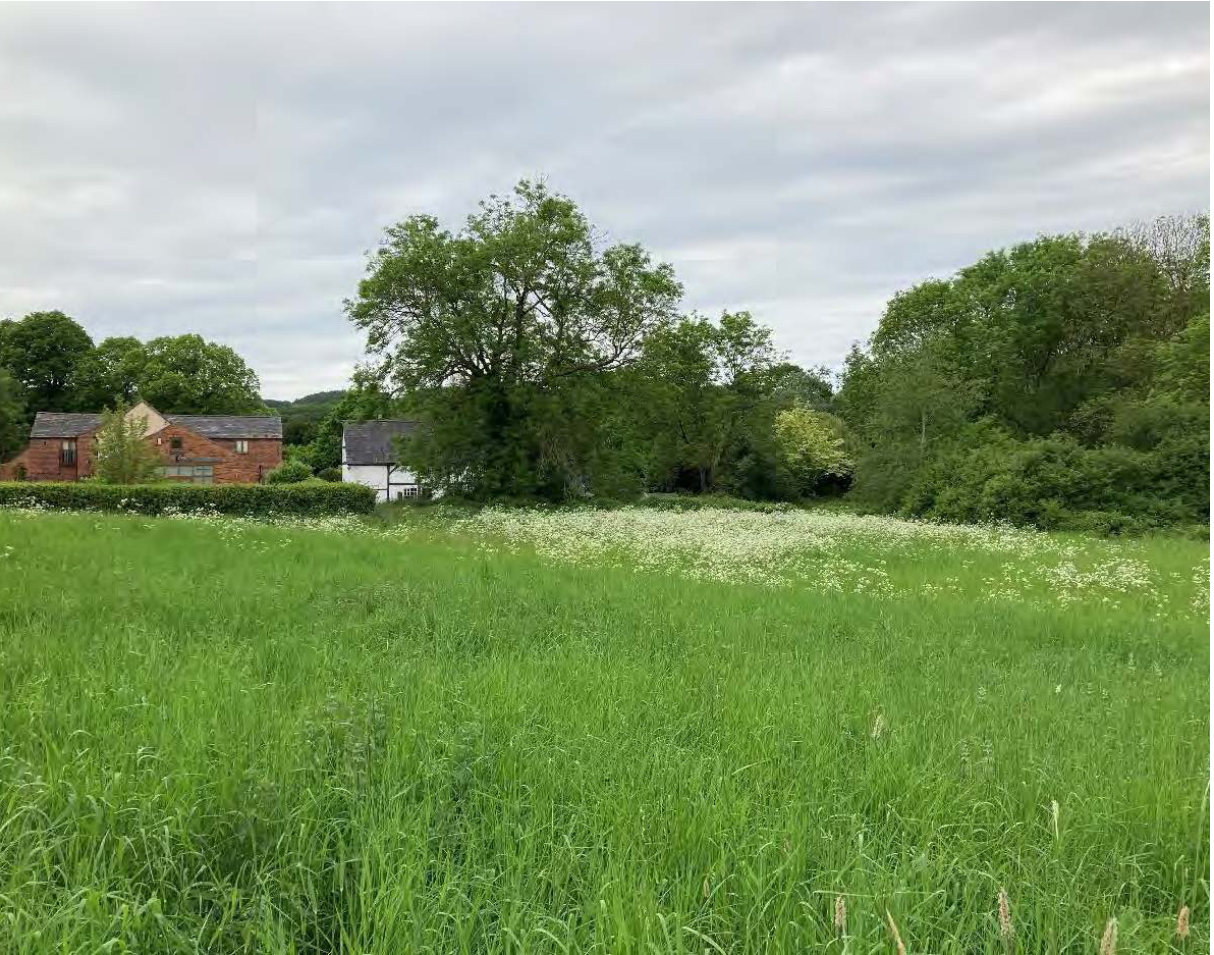
View of rear elevation of Burleigh Farmhouse and adjacent outbuilding (No. 231a) from site to south-west
