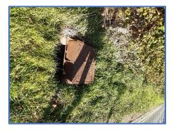
There is a large service cover which will fall within the proposed footway. The metal service cover may pose as a slip hazard for pedestrians particularly during wet conditions.
