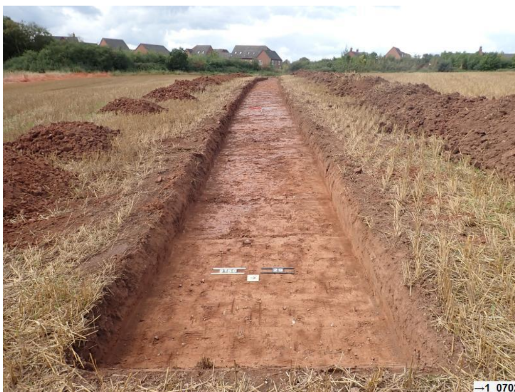
Plate 40: Trench 29 overview, looking west. Scales = 1m
