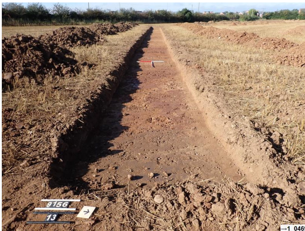
Plate 23: Trench 13 overview, looking west. Scales = 1m.
