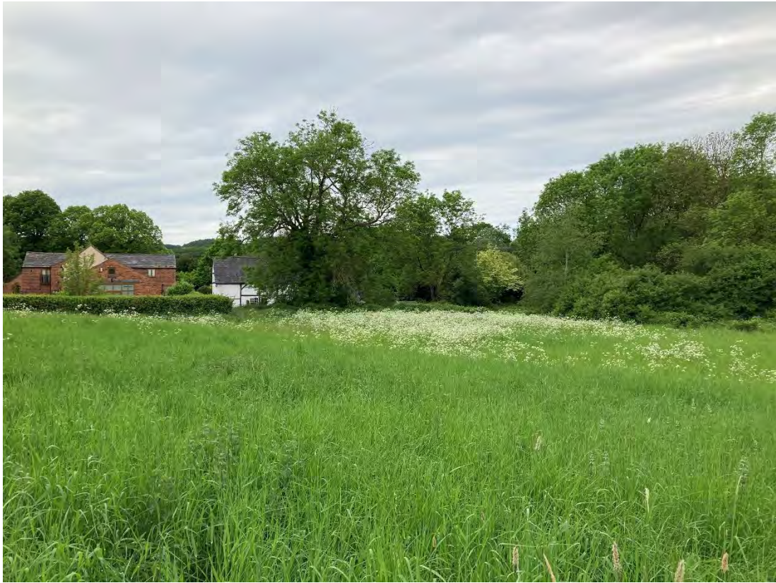
Plate 5: View of rear elevation of Burleigh Farmhouse and adjacent outbuilding (No. 231a) from Site to south-west
