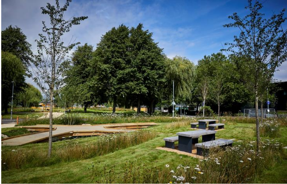
Plate 24: West Gorton Community Park has three distinct design zones, a woodland, a meadow, and a community plaza. Underlying all these areas are water management design features, including a series of swales, raingardens, and bio-retention tree pits. Credit: Groundwork
