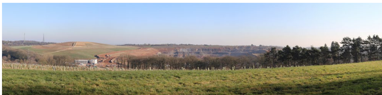
View of Bardon Hill Quarry
