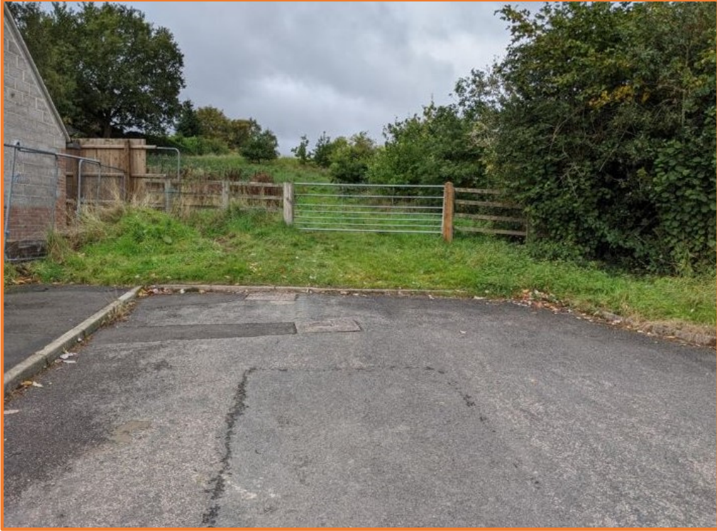
Photo of adopted drainage network in Leconfield Road adjacent to site entrance.
