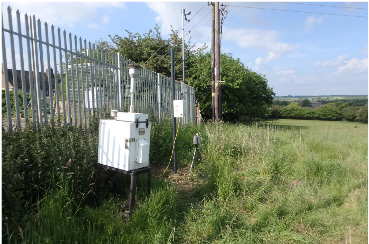
Figure 5: On-site Partisol 2025, Turnkey Osiris and CBC Partisol 2025 beyond, Stn 9 (Hawcliffe Road, Mountsorrel Quarry). A portable PM 10 monitor is also shown (see text for details)
