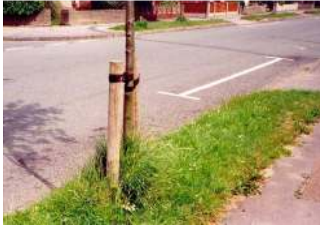
Unacceptable roadside verge maintenance
