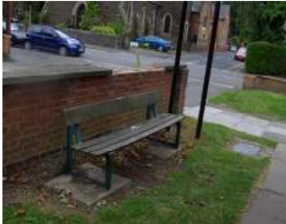
Unsatisfactory, poorly maintained green space furniture which is rusting and rotting
