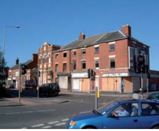
Corner of Leicester Road & Barrow Street
