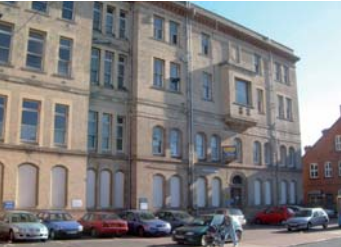
No 56 Baxter Gate: Former Hospital building
