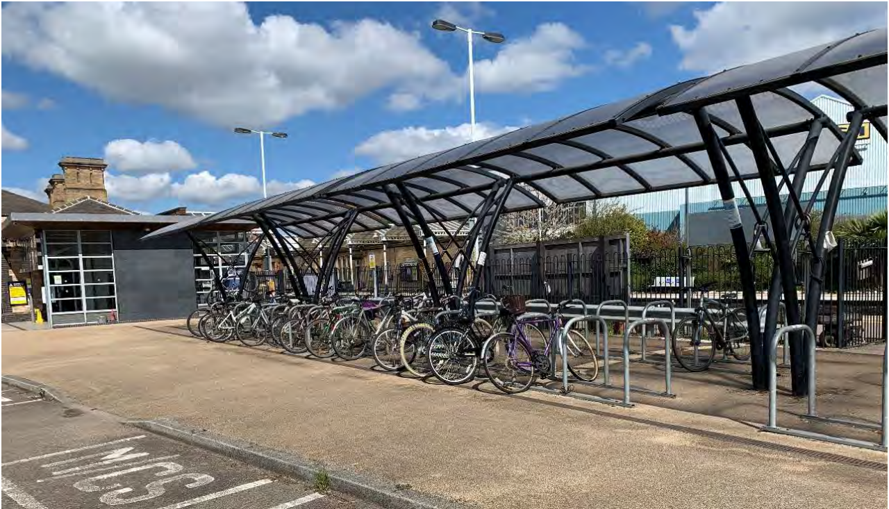
Figure 3-8: Covered cycle parking at Loughborough Station
