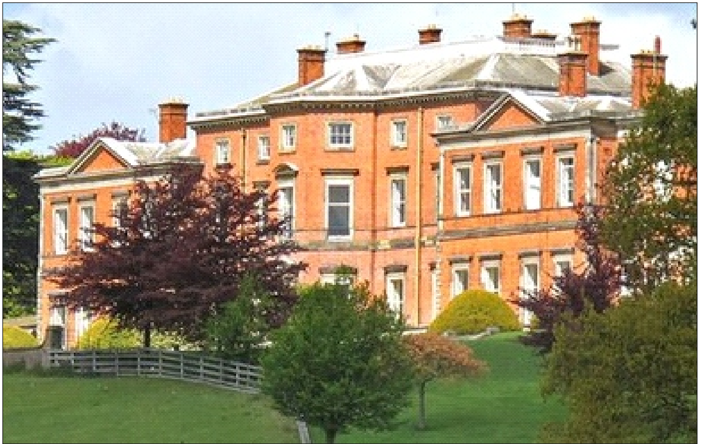
Fig 15 Upper - Preswold Hall (II). Lower - Stanford Hall (II)
