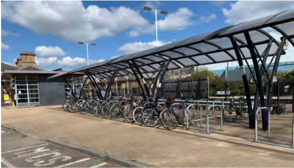
Figure 5-2: Covered cycle parking at Loughborough Station
