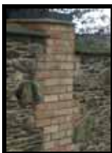
Granite walls with brick posts
