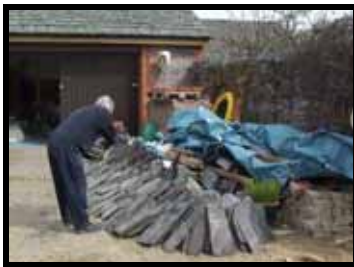
Sorting roof slates
