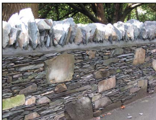
Newly built dry stone wall, Brand Hill
